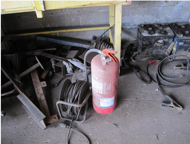
Extinguisher out of place without maintenance
