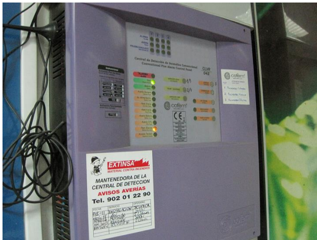
Control panel with errors
