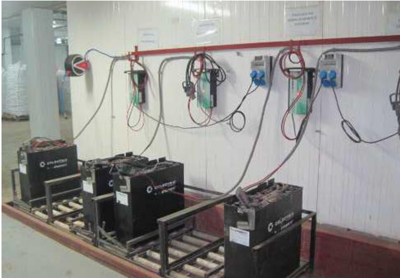
Forklift battery chargers on combustibile sandwich panel
