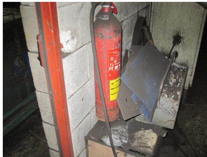
Extinguisher blocked by waste
