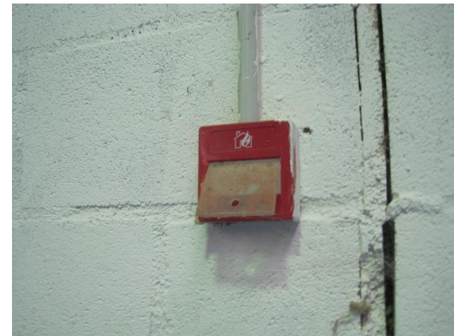
Damaged call point
