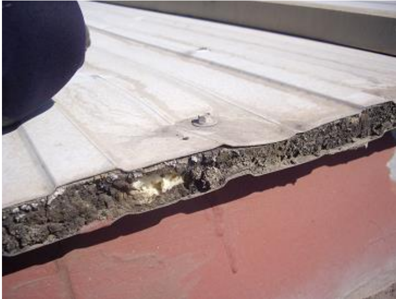
Sandwich panel with combustible insulation (PUR)
